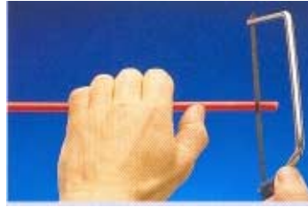
1 . Saw the cable to produce a square end.
