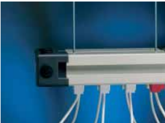
The distribution box can be suspended on drop rods utilising Caddy Clips.
