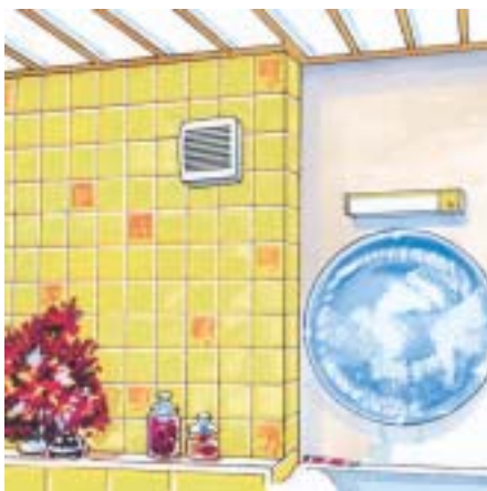
A typical wall mounted fan
