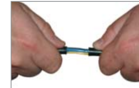
Slide conductors out of sheath.
